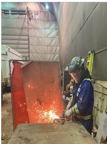
Figure 2-5 Use of Welding Screen
