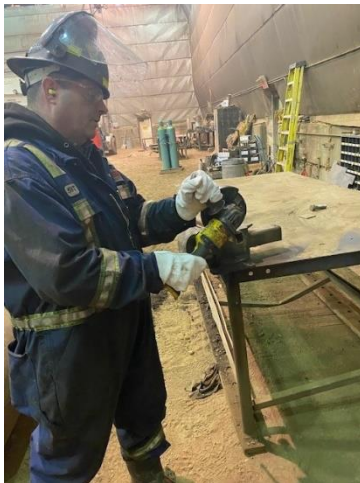
Figure 2-0 Incorrect Cutting Technique
